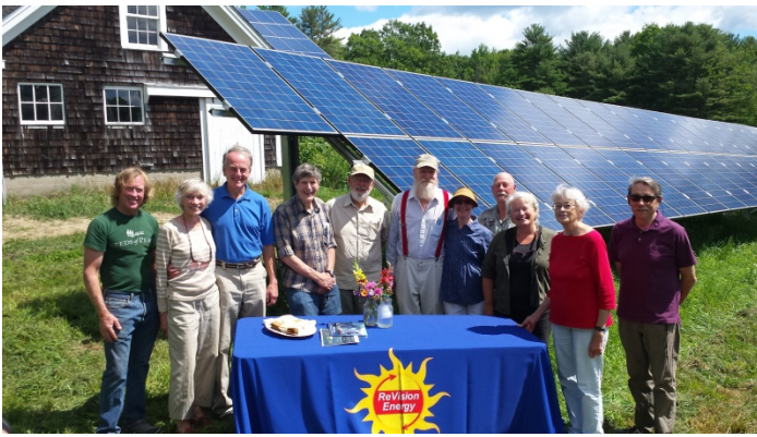
A green bank would support deployment of solar energy projects, such as this community solar farm in Edgecomb, Maine, to help the state catch –up to neighboring states and the rest of the country. (Revision Energy)
